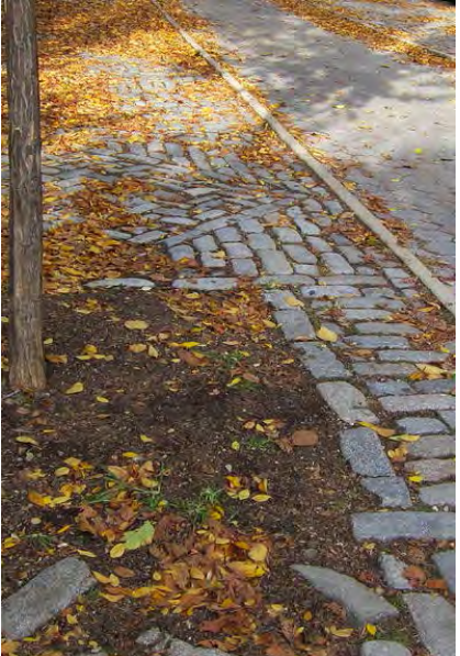
Granite Block Paving
