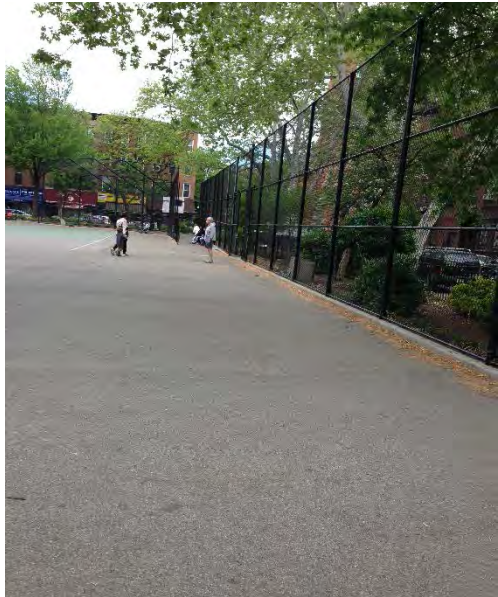
Full Depth Asphalt
